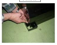
4. Hang the (4) upright trim sections at each corner. Insert the hooks at the top end into the slots in the lid while guiding the bottom into the trim cup mounted on the base near the floor (fig E).
