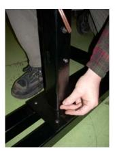
Attach the handle to the rear of the main pole with (2) 10-32 X ½" (L) screws about 12 inches below the top of the pole on the rear side.
