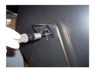
2.Assemble the support tubes to the sign box. Start by feeding the wire leads from the sign box through one of the tube supports.
